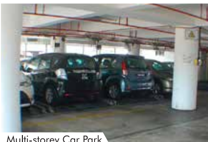
Multi-storey Car Park
