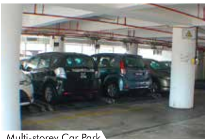
Multi-storey Car Park
